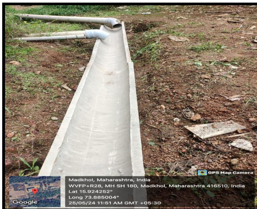
Effluent Treatment Plant
